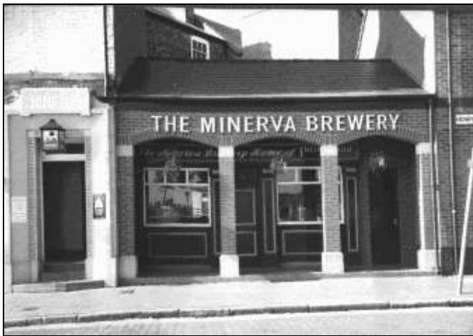
Figure 7 The Minerva Brewery on the site of the Vaults
